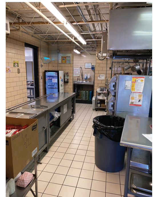
Food Service Condition
