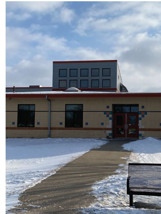
Typical exterior condition
