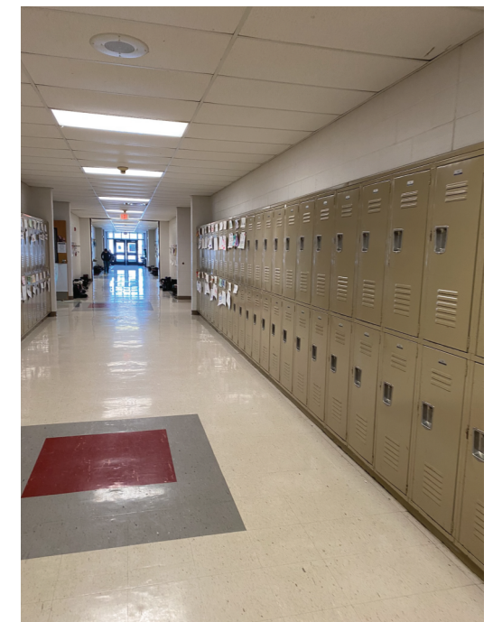
Typical corridor condition
