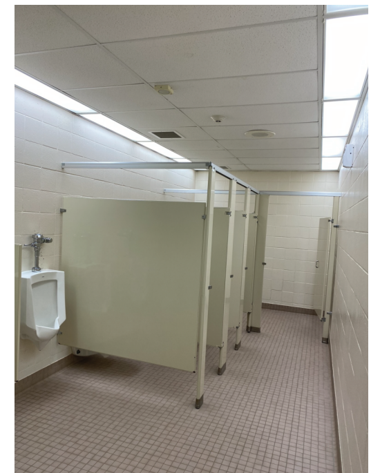
Typical bathroom condition
