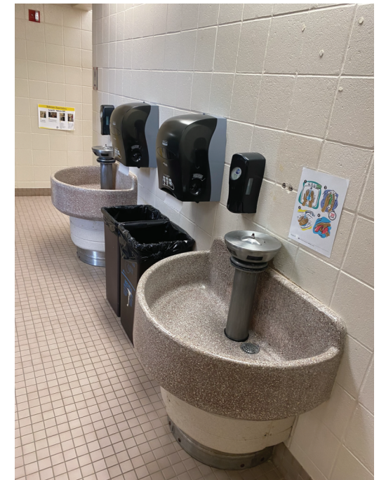
Typical bathroom condition
